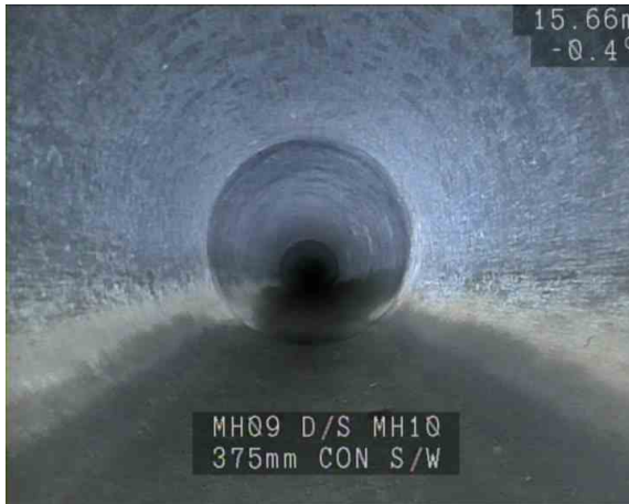
_390ca381-15d0-418f-a45c-e2b560419aa3.jpg, 00:03:03, 15.66 m General Condition photograph
